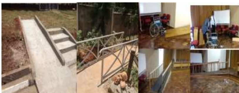
Ramps and Rails across the Compound
